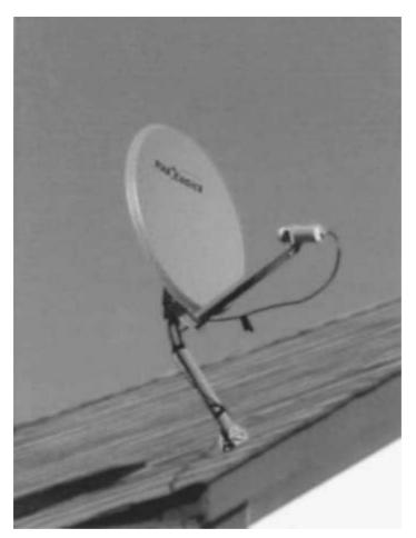
Figure 16.6 A typical DBS antenna installation.
