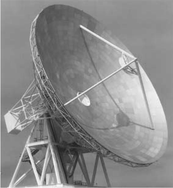
**Figure 8.7** Standard-A (C-band 6/4 GHz) 32-m antenna.
