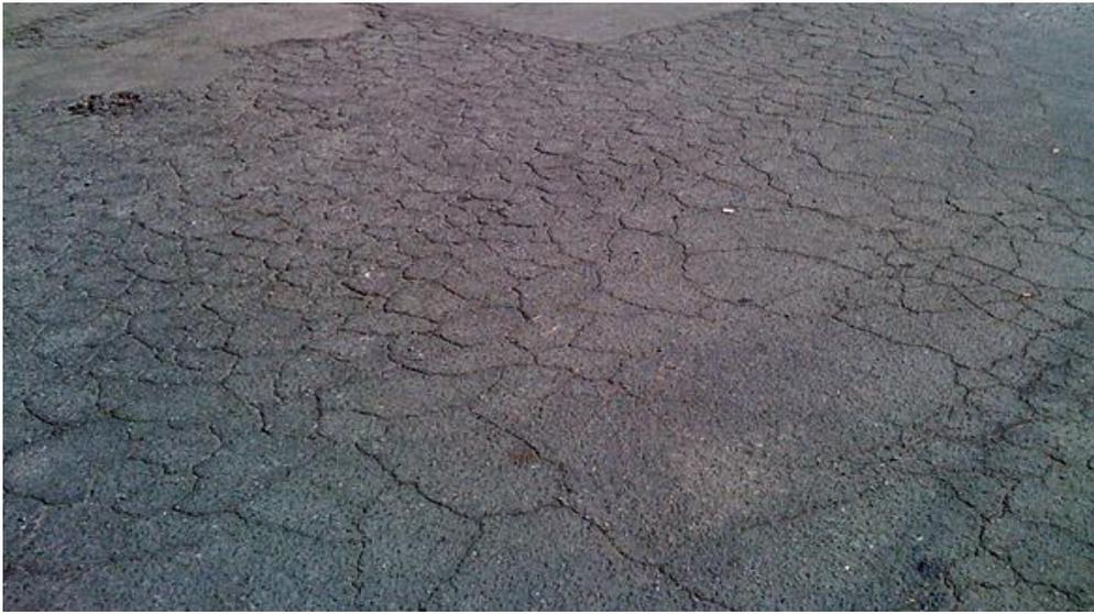
Fig. Alligator Cracking
