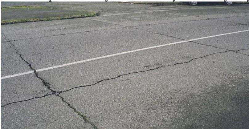
Fig. Joint Reflection Cracks
