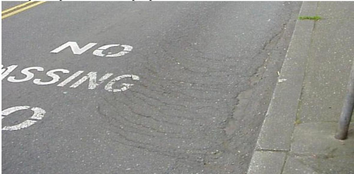
Fig. Slippage Cracks
