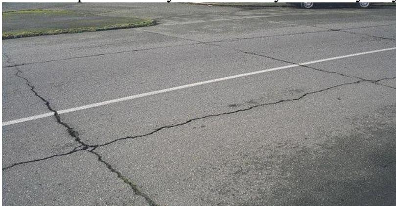
Fig. Joint Reflection Cracks
