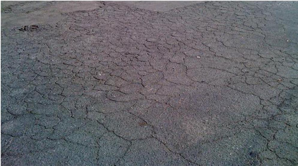
Fig. Alligator Cracking
