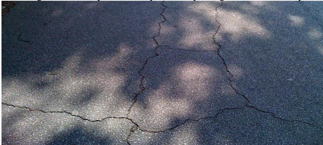
Fig. Block Cracking
