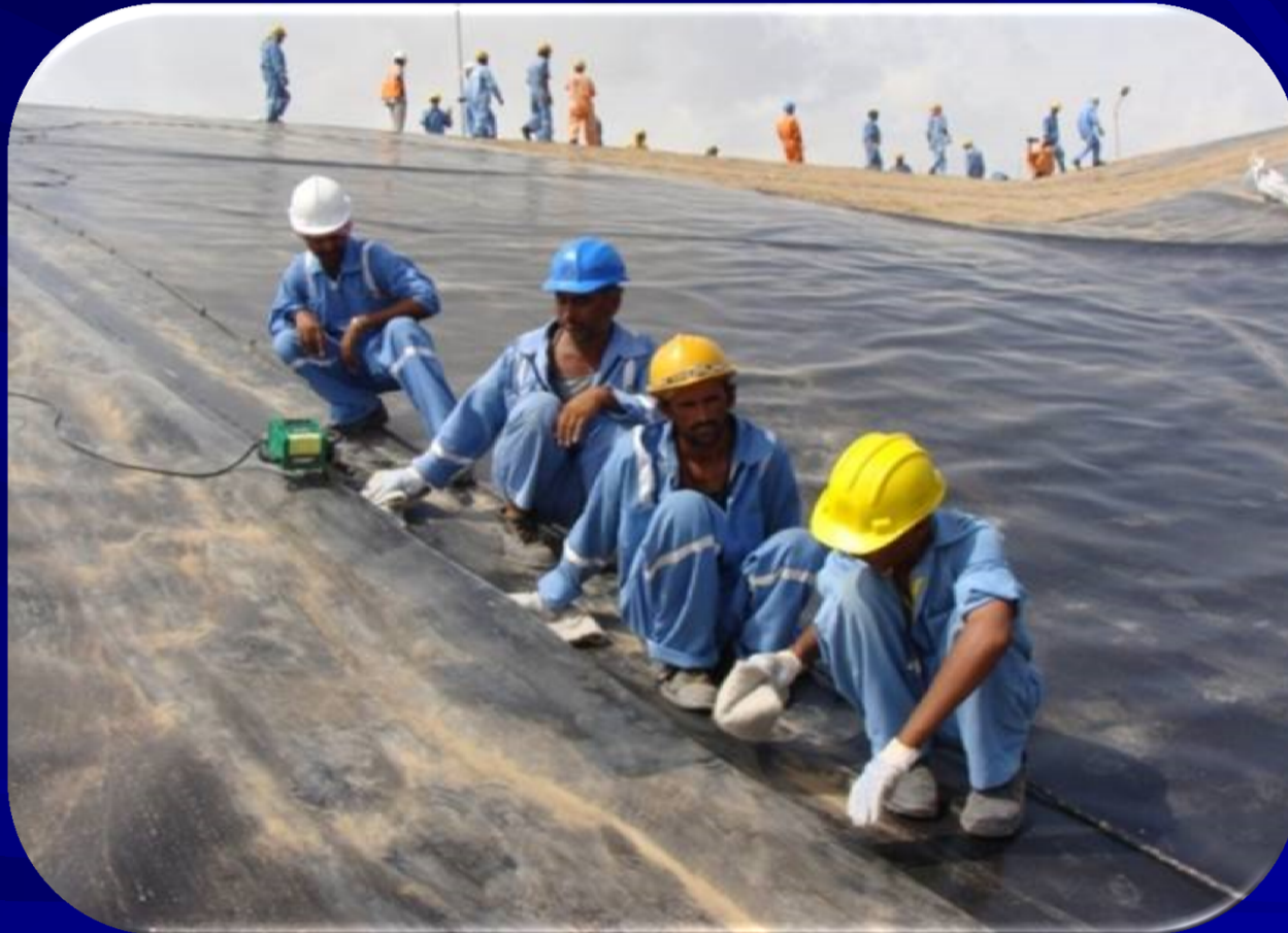
Installation of Geomembranes
