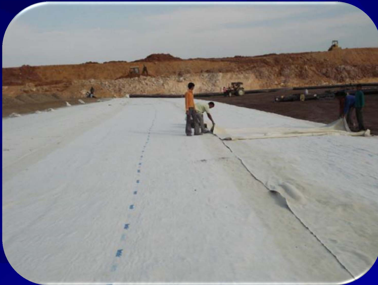
Installation of GCL
