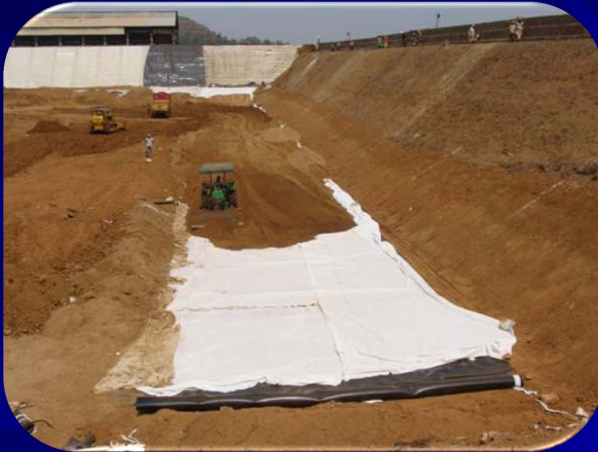
Geomembrane and drainage installation
