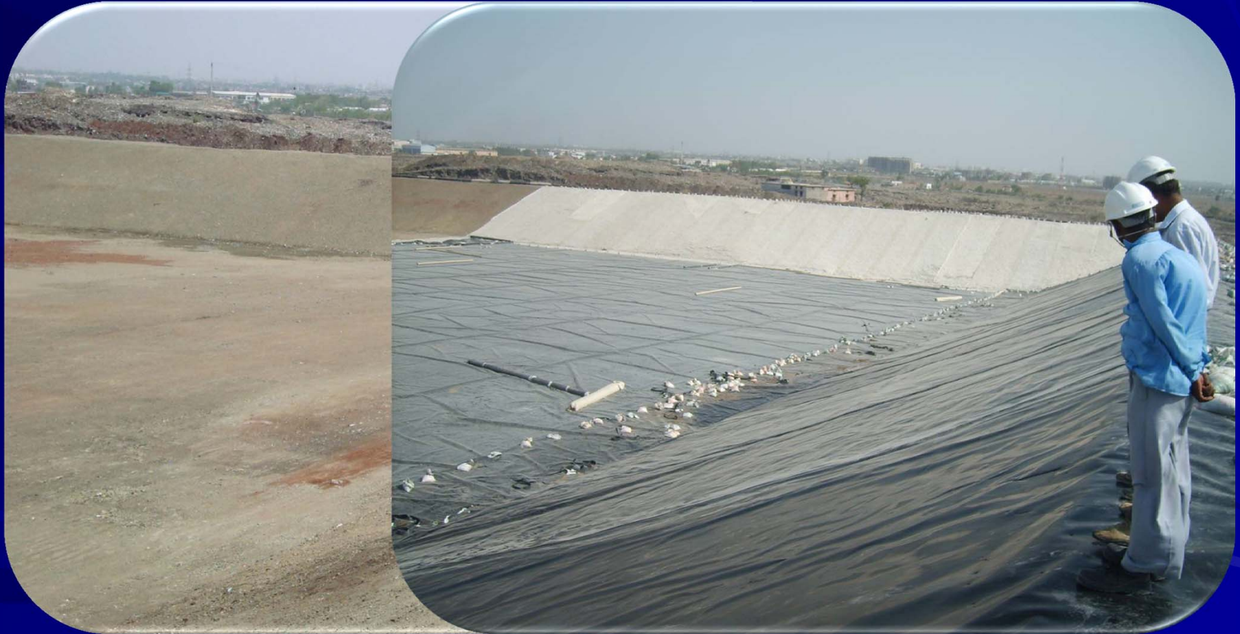
Installation of GCL
