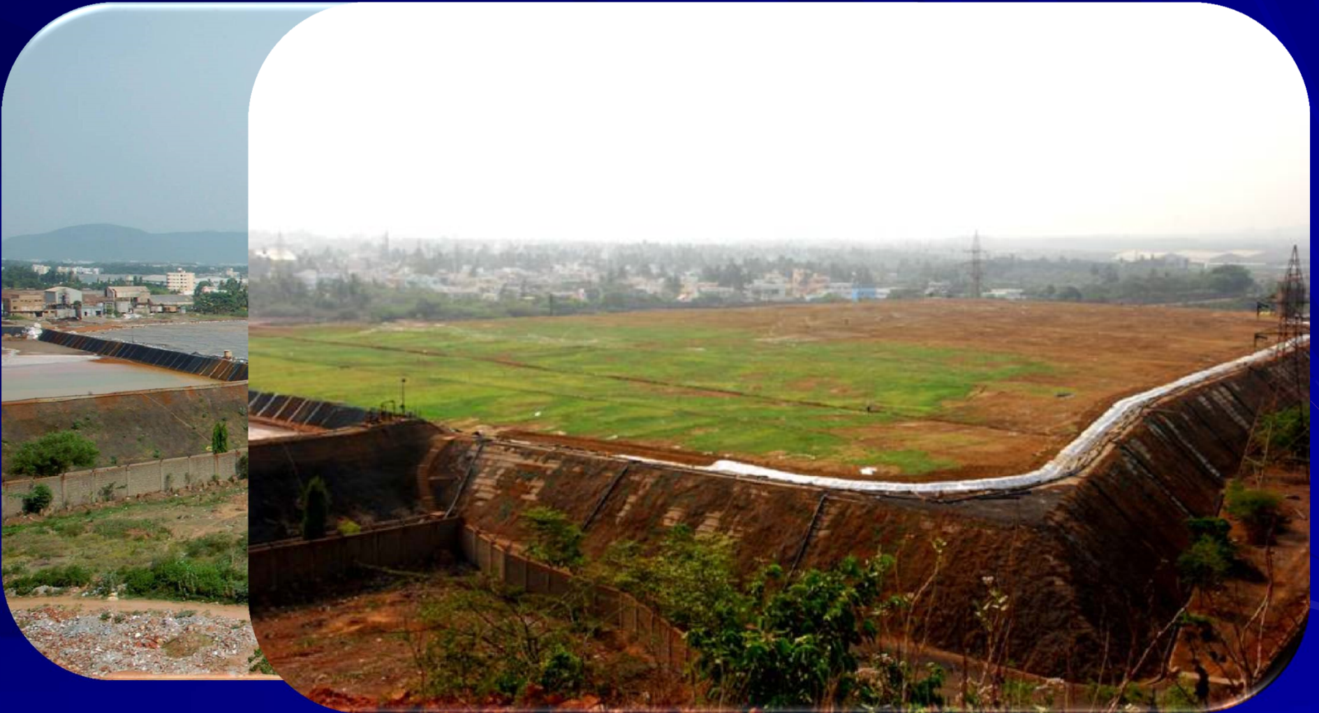
Installation of Geomembrane as Closure
